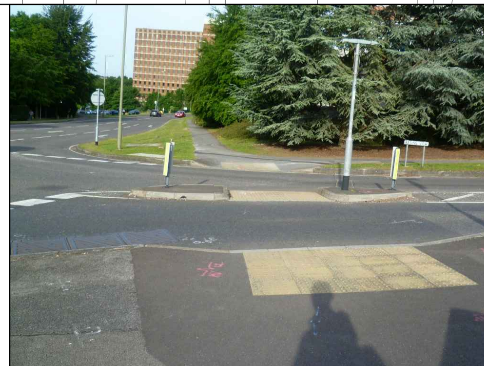
EXAMPLE OF UNCONTROLLED CROSSING Vehicles have priority, dropped kerbs and tactile paving provided.
