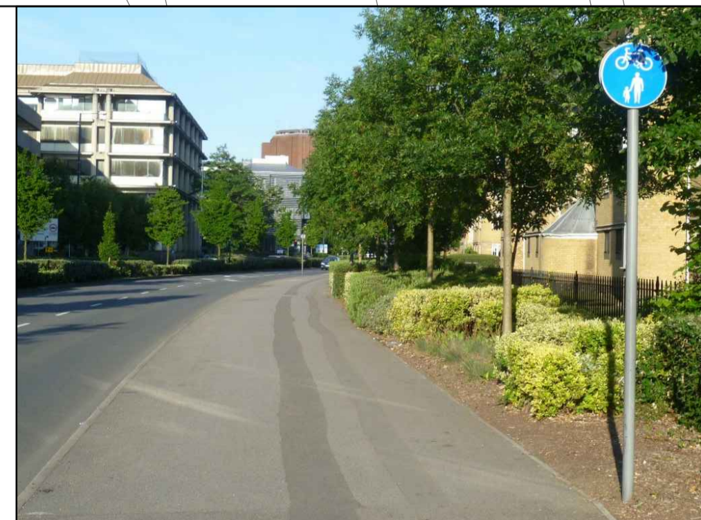
EXAMPLE OF SHARED USE CYCLE PATH No segregation between cyclists and pedestrians.
