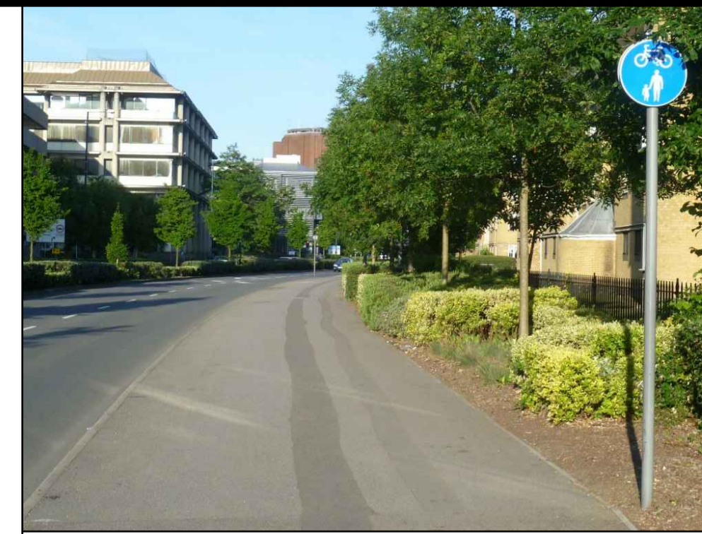
EXAMPLE OF SHARED USE CYCLE PATH No segregation between cyclists and pedestrians.
