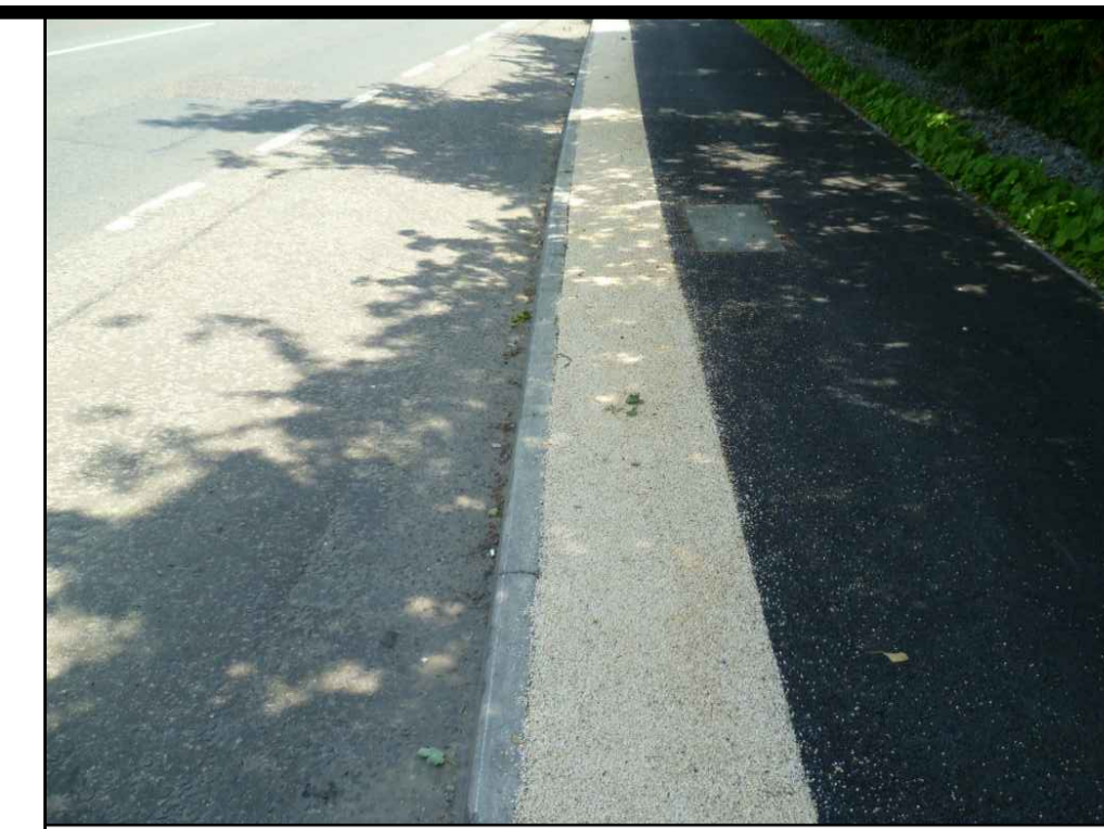
EXAMPLE OF PAVED MARGIN Separation strip between road and cycle path.
