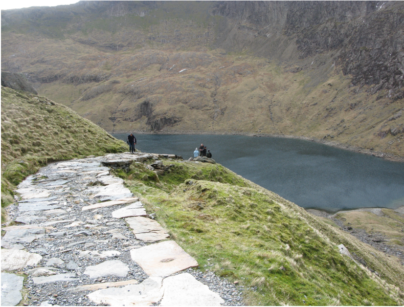
image 3: public footpath repaired after erosion by walkers
